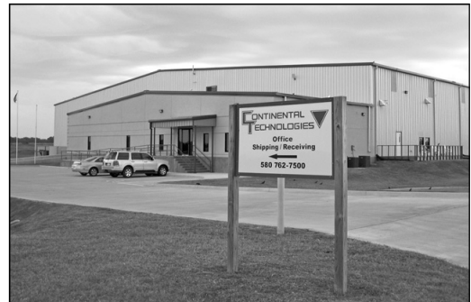
Continental Technologies, 2405 Sykes Boulevard, is one of the new premiere industries to locate in Ponca City. The building, previously known as "Bob," was constructed by the Ponca City Development Authority as a "spec building," to attract industry to town. (News Photo by Louise Abercrombie)
